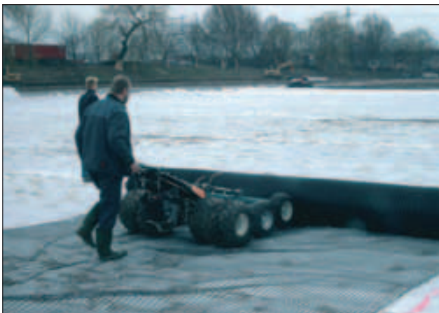
Installation of Fortrac® geogrid
