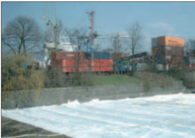
Installation of Stabilenka® geotextile
