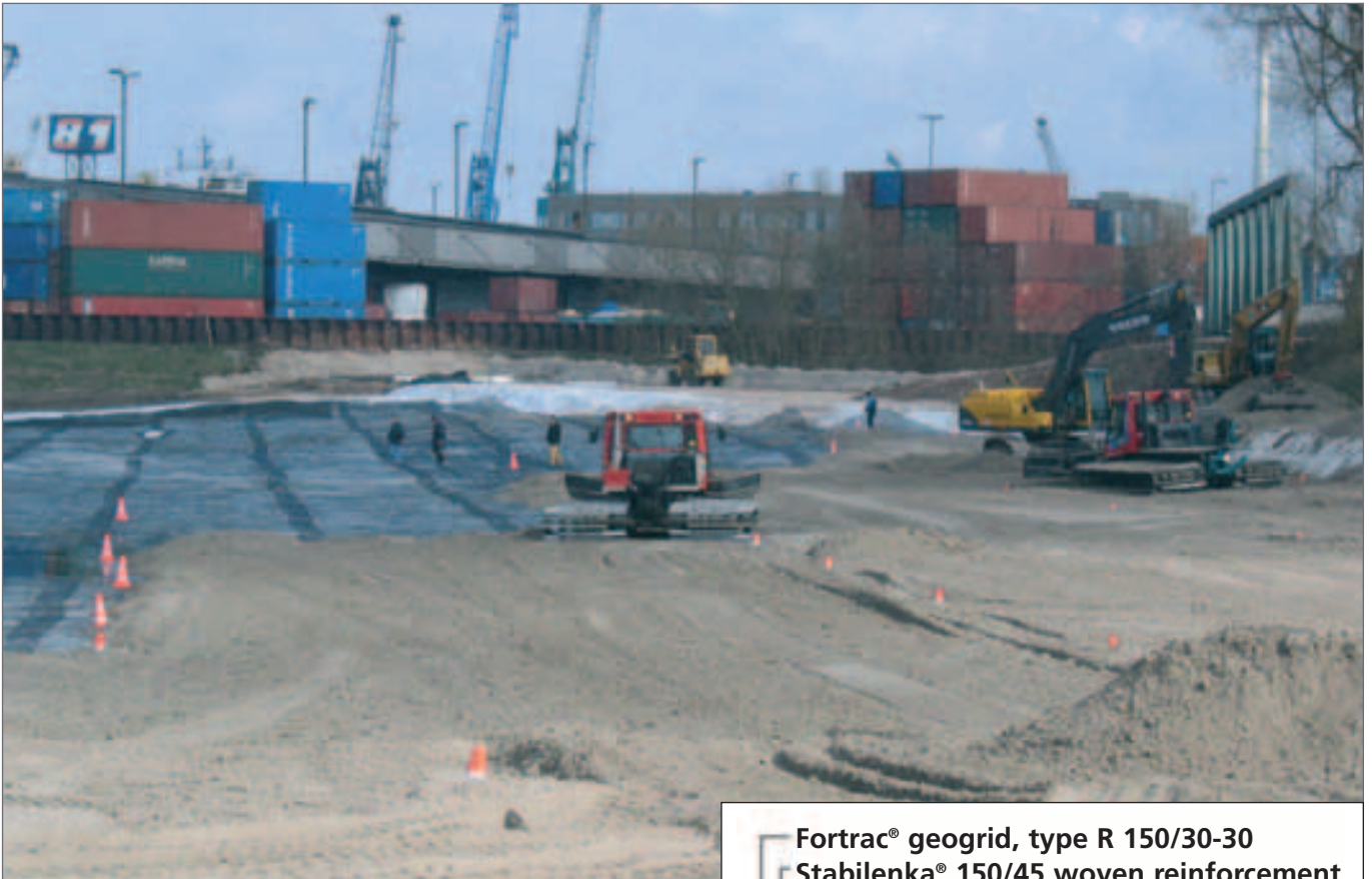
Overview: Rodewisch Harbour during the placement of the initial sand layer
