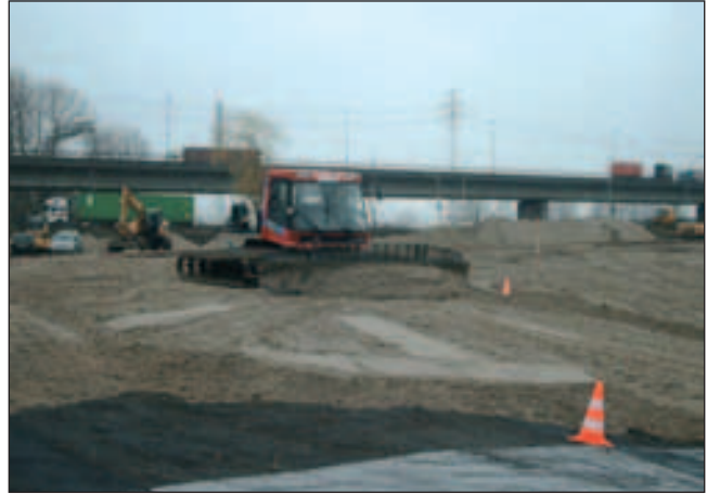
Spreading sand-fill over geosynthetic reinforcement
