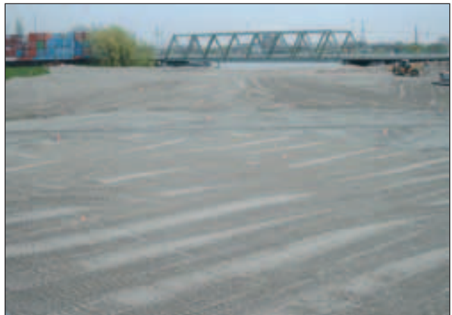
Rodewischhafen after ground preparation
