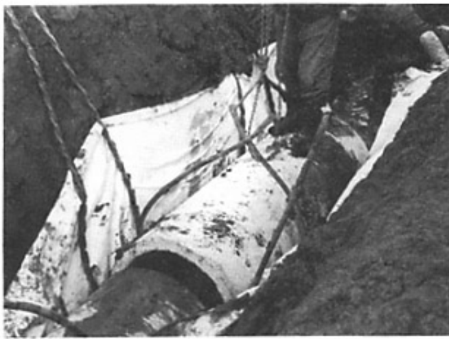
Photo 1. Pipes during geotextile placement.
