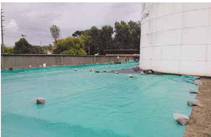
Tank Farm Petrobras Dock Sud - Avellaneda, Bs. As.
